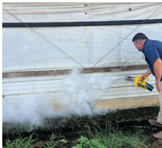
Smoke testing a curtain-sided house to identify air leaks.
