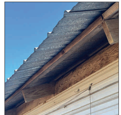
Traditional 2 x truss tail purling
