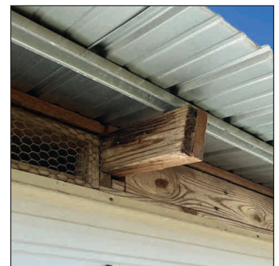
Replaced metal purling and truss tail repair
